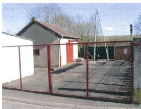
Station de Lauvallières
